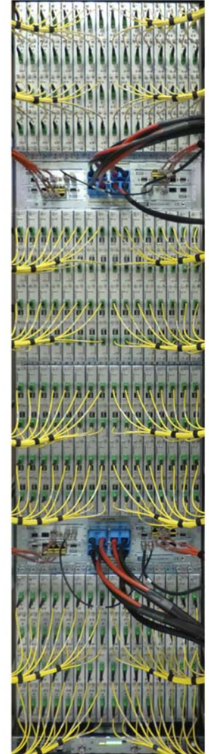
EQXM Rear View MTP Rear Plate wired for 1152x1152
